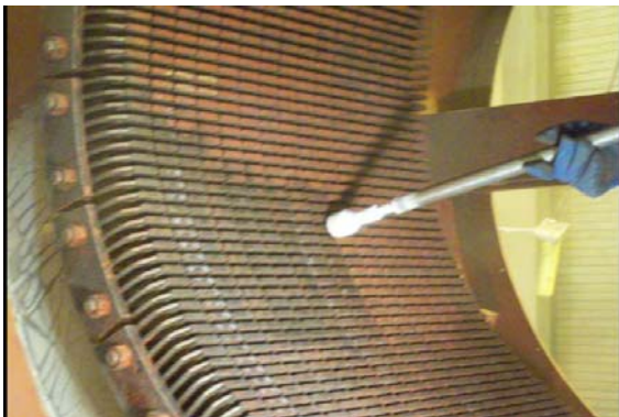
The NitroJet proved to be very efficient in removing paint and fiberglass material from the motor.
