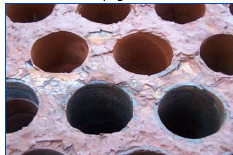
Example of a tube sheet. The bottom row has been cleaned.
