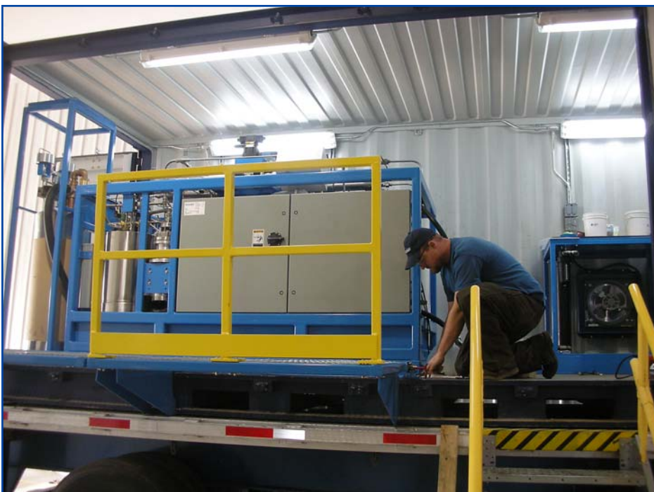
Bryan Gillihan works on Conco's mobile system.
