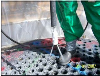
The rotating nozzle is used to clean the tubes of the heat exchanger.
